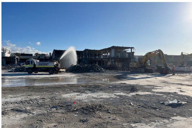
Demolition of the centre continues
